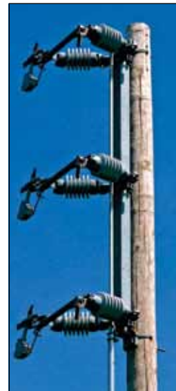
Phase-over-Phase Mounting
