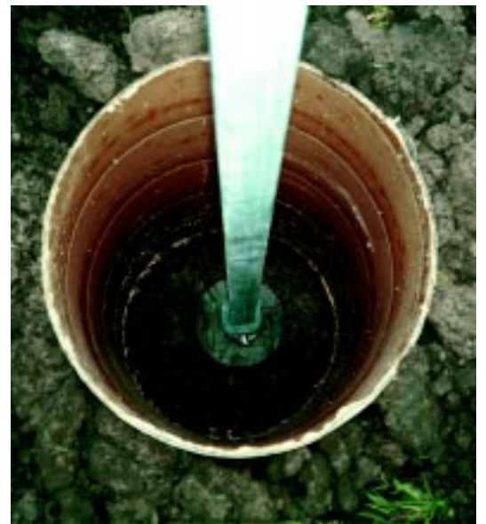
Displacement plates form grout column to design depth
