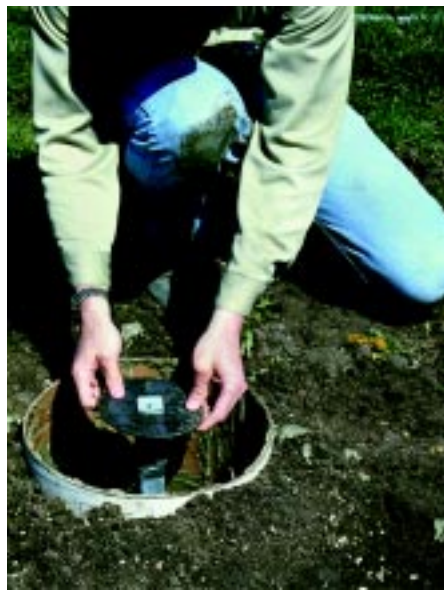
Displacement plates form grout column to design depth
