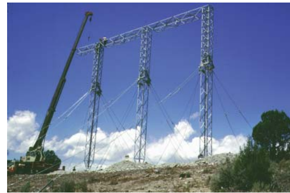
Total Transmission Support: Job-specific teams Chance helical foundation and guy anchors plus top and bottom guy deadends in Chance Adjust-A-Grip® and Fargo brands.
