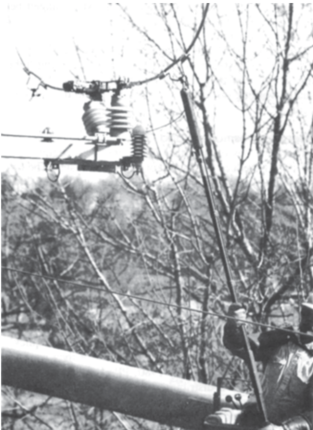
Fig. 3. Linemen must use hot-line tool to energize any arrester.
