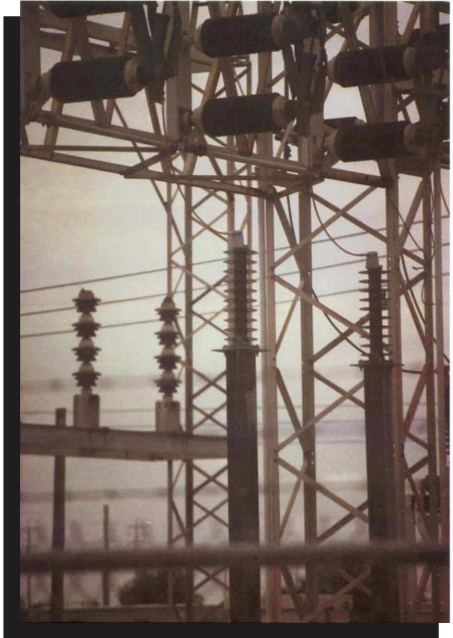
Lightweight PVN arresters were easy to install.
