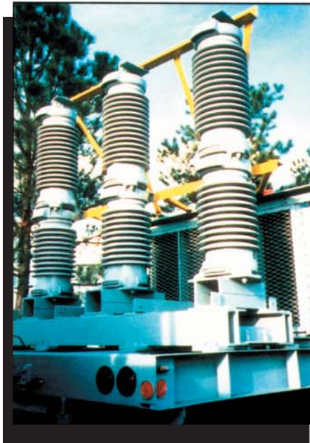
Old silicon gapped arresters.
