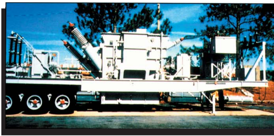
Mobile sub after retrofit.
