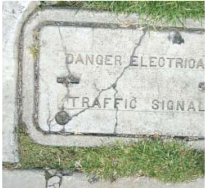
**A cracked cover is a failed cover because its design performance capability has been compromised.**
