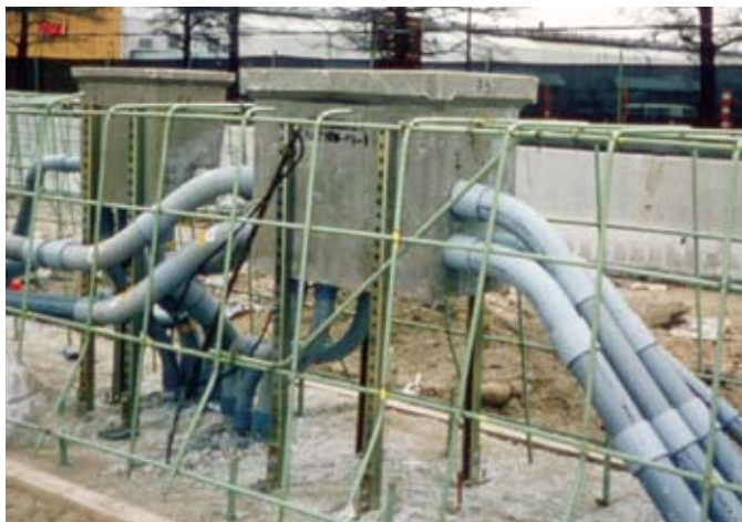
QUAZITE® enclosures can be imbedded in median barriers to serve as signal and lighting junction boxes.
