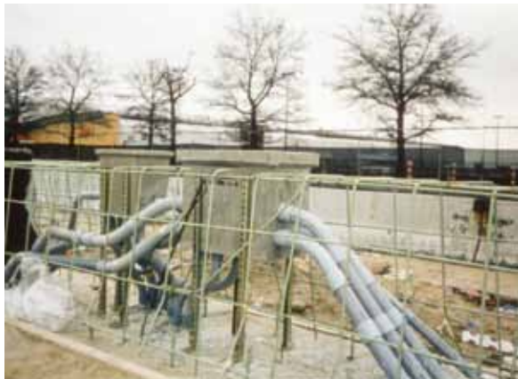
QUAZITE® enclosures can be embedded in concrete highway median barriers for signal and lighting junction boxes.
