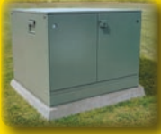
Pad-Mounted Switches
