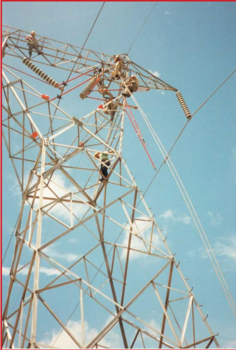
**Costa Rica, left, a maintenance crew gets on-the-job training from Chance Hot-Line Tool Specialists atop this 230 kV tower. The V-string of insulators is supported in an Epoxiglas® cradle positioned by wire-tong hot sticks.**
