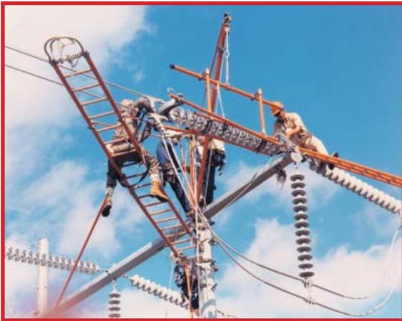
***Above, isolated from the ground plane by sitting on Epoxiglas insulated ladder, conductive garments permit "barehand" work directly on the hardware of this energized transmission line.***
