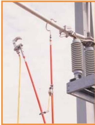
***Teamwork safely lands the large clamps required to ground substation buswork. Shepherd-hook assist stick features a sheave with lift line to manage control.***
