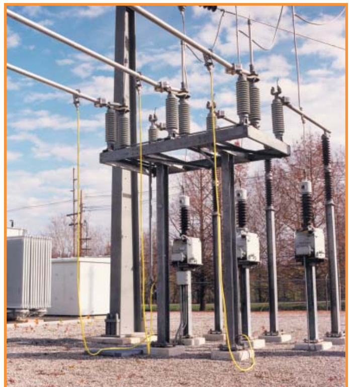
For optimum efficiency, locate ball studs at serviceable heights on substation legs. As available as any option, these custom-made substation cable sets each combine a bus clamp on one end and a socket-type on the other.
