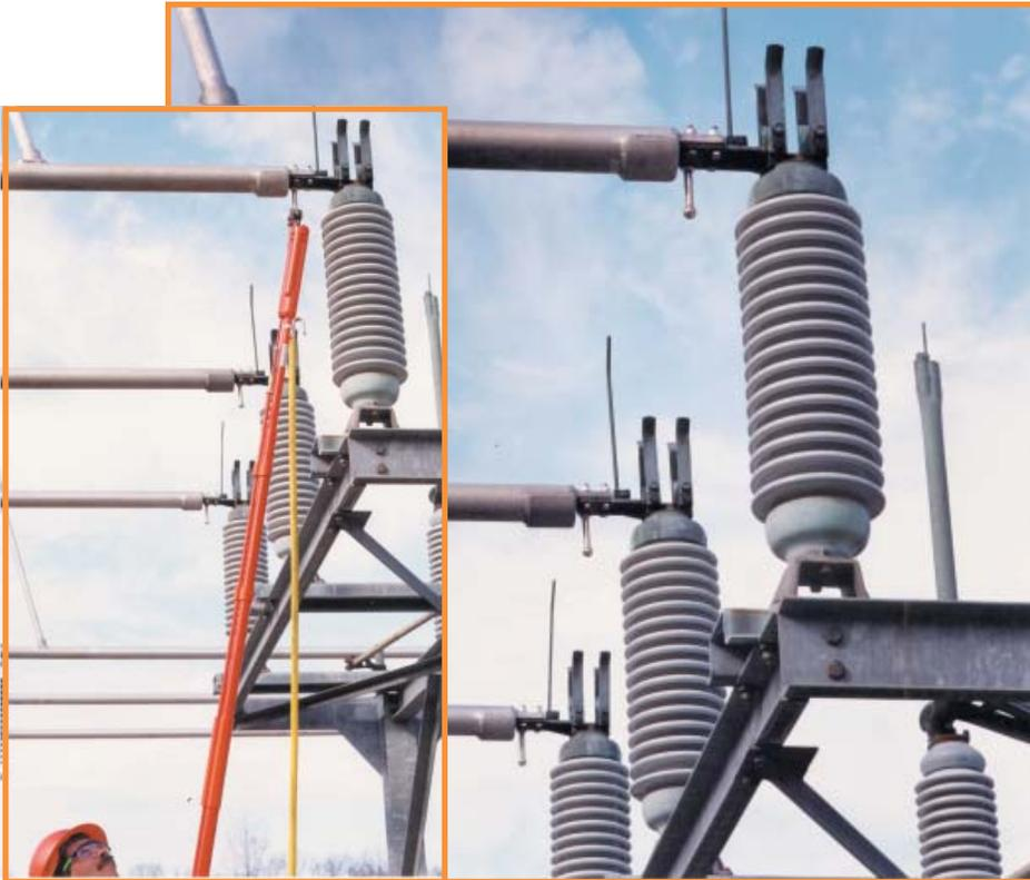
**Socket clamps and ball-stud connectors team up for easy attachment of grounds from most any approach angles using a standard clampstick.**
