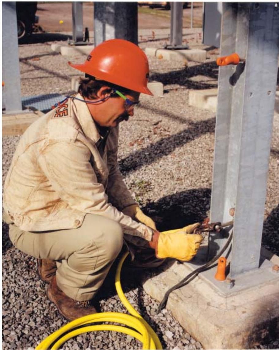
***Permanently installed ball-stud terminals accept socket-type clamps for convenient interconnection to substation ground grid. Optional covers snap on the ball studs to reduce corrosion and contamination when not in use. The covers are made of the same nonconductive thermoplastic elastomer material as Chance cover-up line hose .***
