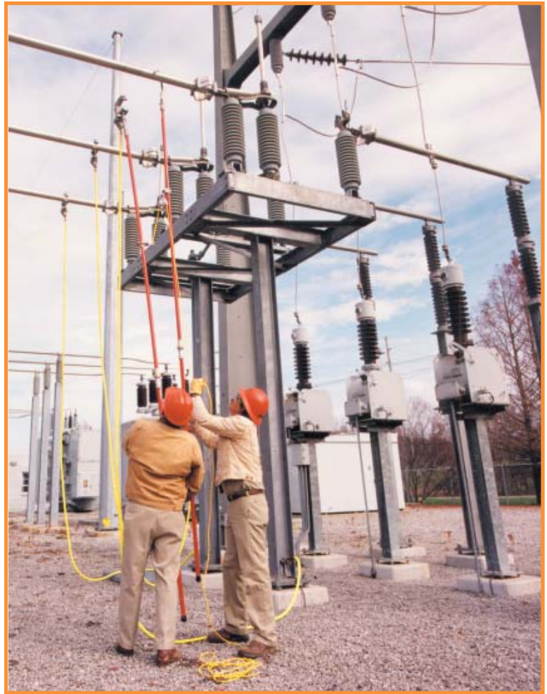
For optimum efficiency, locate ball studs at serviceable heights on substation legs. As available as any option, these custom-made substation cable sets each combine a bus clamp on one end and a socket-type on the other.
