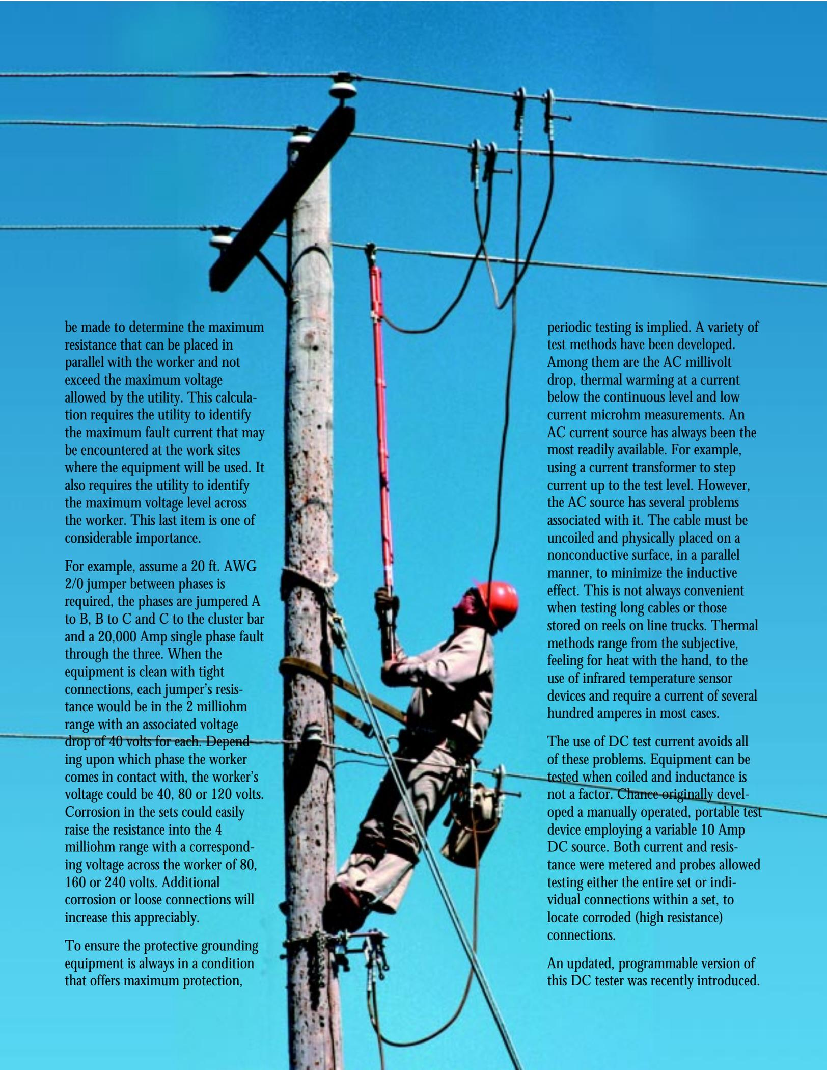
be made to determine the maximum resistance that can be placed in parallel with the worker and not exceed the maximum voltage allowed by the utility. This calculation requires the utility to identify the maximum fault current that may be encountered at the work sites where the equipment will be used. It also requires the utility to identify the maximum voltage level across the worker. This last item is one of considerable importance.
