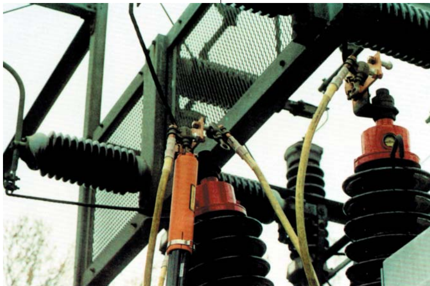
New system makes grounding easier. Ball studs mounted back-to-back on copper plate add convenience for placing socket clamps of phase-to-phase ground leads. Torque-controlled clampstick head ensures proper tightening.
