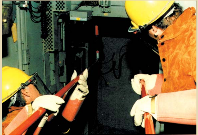
Plant electricians use Chance phasing tool to confirm absence of line voltage prior to applying grounding cables.
