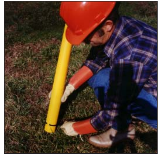
Guy marker covers three-bolt suspension clamp and anchor rod to allow full coverage to the ground.
