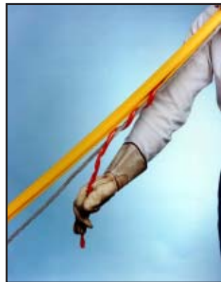
Apply pigtail by wrapping around guy.
