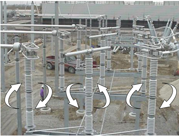
Three rotating insulators provide smooth and reliable operation.
