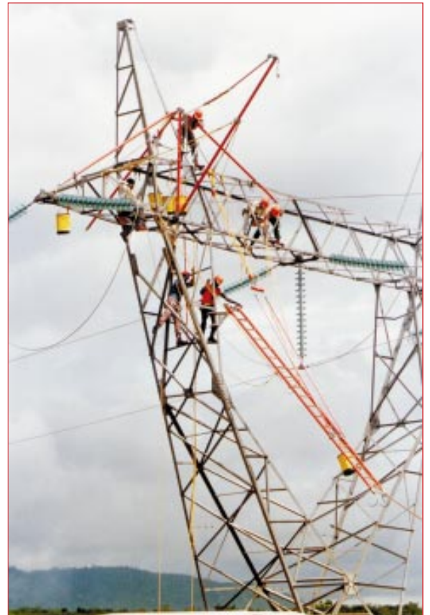
Tanzania, above, crew raises hook ladder while learning cargo-boom method for live installation of deadend insulators on 230 kV free-standing tower.
