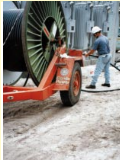
Starting to unreel cable for pull.
