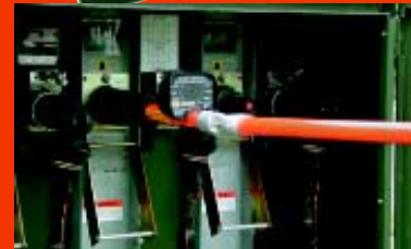
ARVI holds reading for voltage-indication tests on switch bushing (above) and cable (at right, using a feed-thru device).
