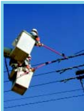
Phasing Tester lets you quickly identify overhead phases and read voltage for Ø-G and Ø-Ø tests.
