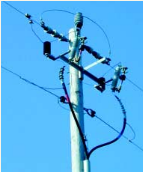
Underground tap application of Chance Electronic Sectionalizers enhances protection coordination and improves utilization of cable ampacity.
