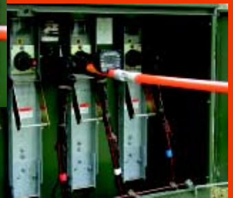
ARVI holds reading for voltage-indication tests on switch bushing (above) and cable (at right, using a feed-thru device).
