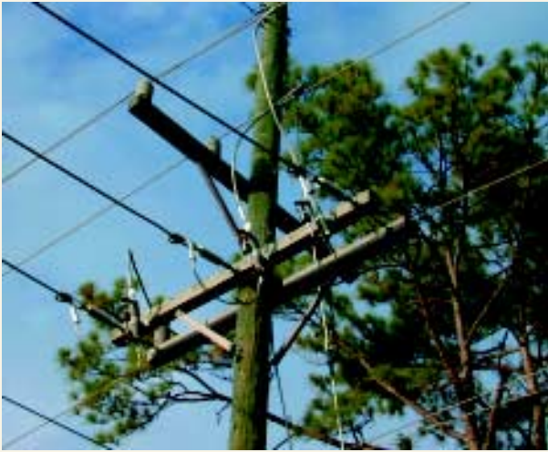
Overhead lateral tap application of Chance Electronic Sectionalizers eliminates nuisance outages.
