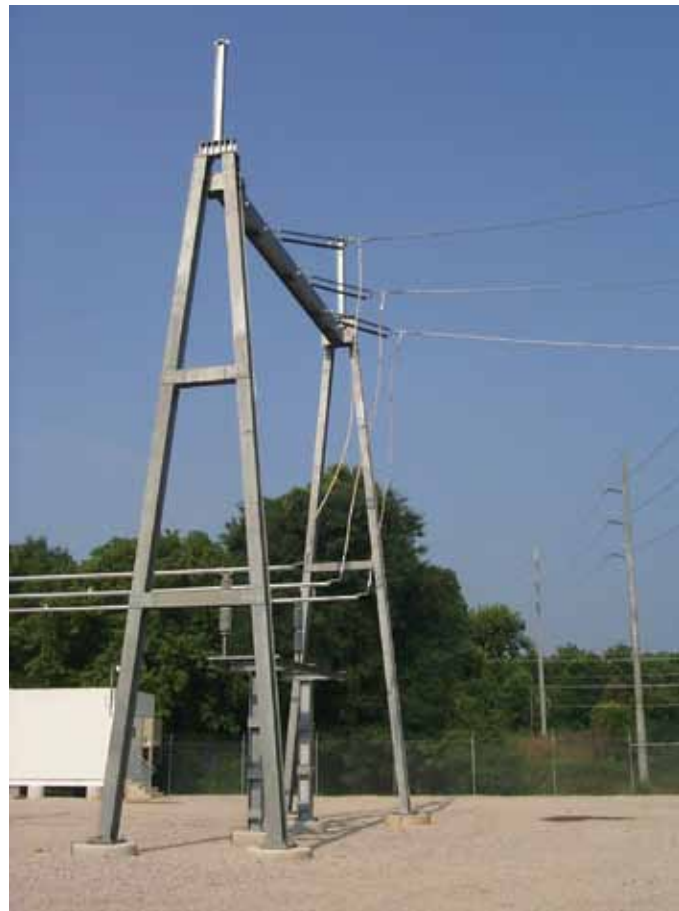
Protecta*Lite is used for all transmission substations. Units are placed in parallel with the string of deadend insulators.
