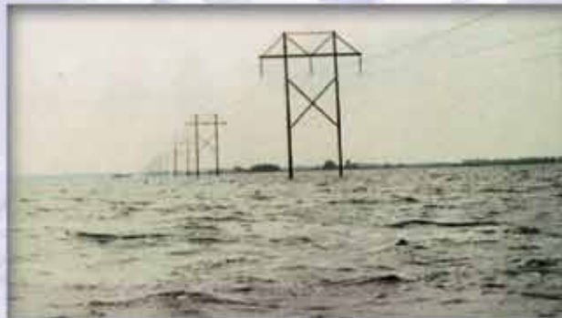
Transmission line in Devils Lake in 1995 at a lake elevation of 1435 ft.
