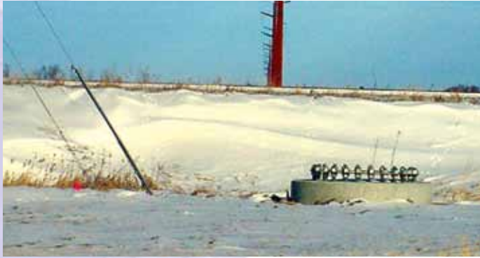
Close-up of foundation prior to setting of 90-ft pole.
