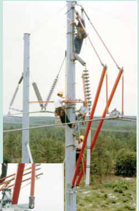
Steel H-frame, 230kV Horizontal-Vee, Bundle Conductor 795 ACSR
