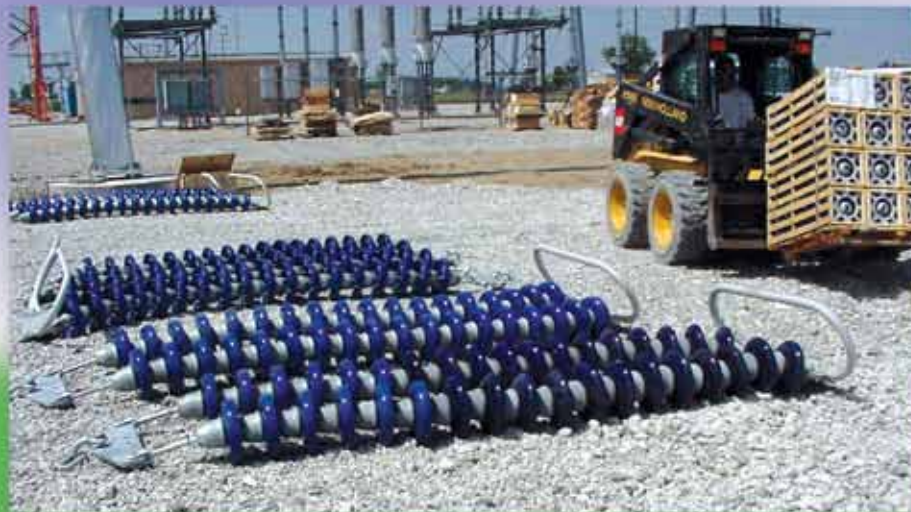
Deadend hardware assembled to deadend insulator strings prior to installation
