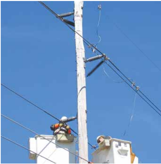
Two PROTECTA*LITE Arresters set; working on installing third arrester.
