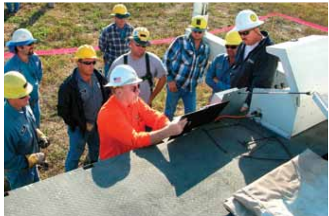
The barehand team learns about monitoring equipment that alerts voltage leakage on the insulated truck boom.
