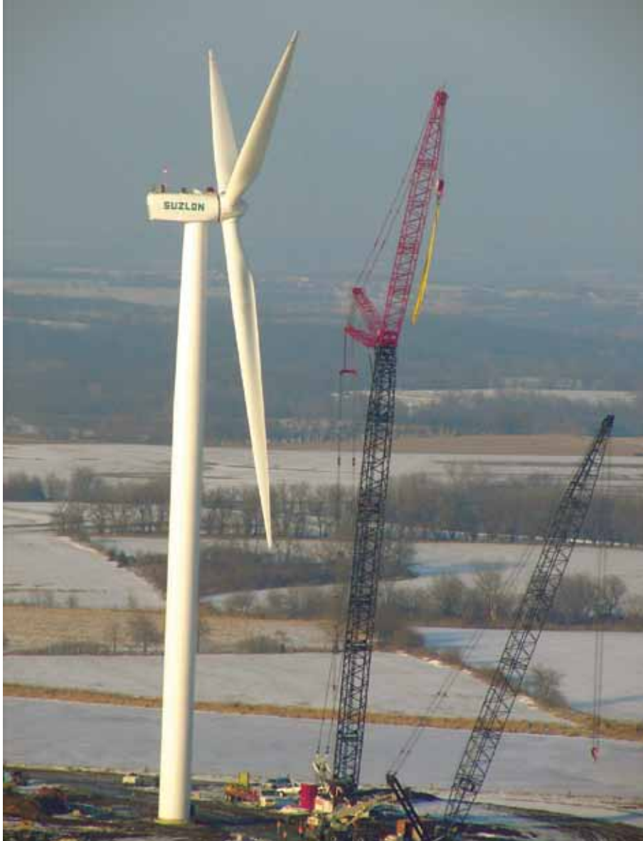
Last wind turbine being assembled.
