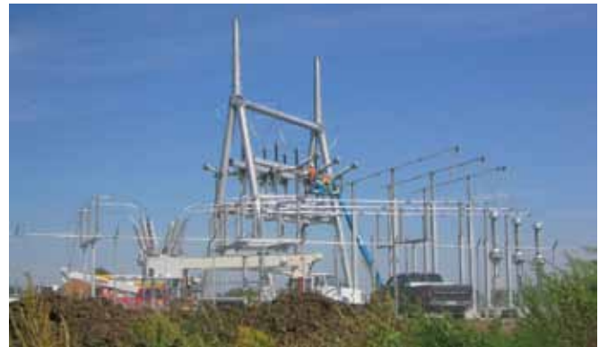
Men working in Gentry Substation assembling one of the 161-kV transmission switches used to isolate one side of the transmission line from the other and to allow the wind farm to feed the transmission line.
