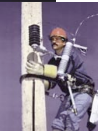
Installing a surge arrester.
