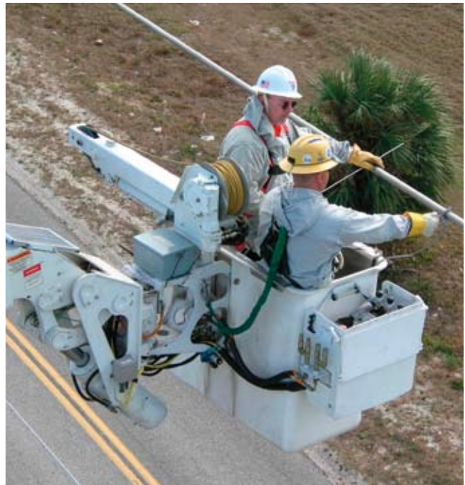
LCEC transmission lineman makes connection to the line with a bonding clamp as instructed by Randy Beckes, Chance® Tool Demonstrator.
